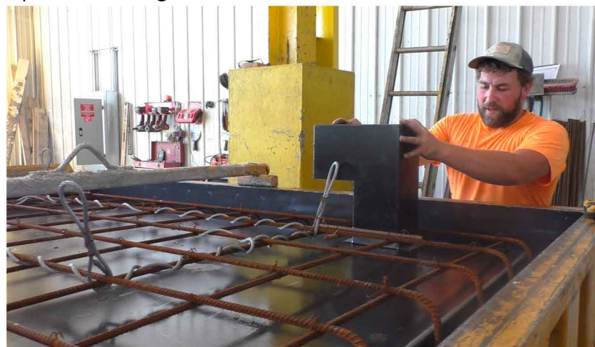
Lucas McAtee points out the ventilation system coming up through the rebar before the concrete is poured to form a storm shelter.
